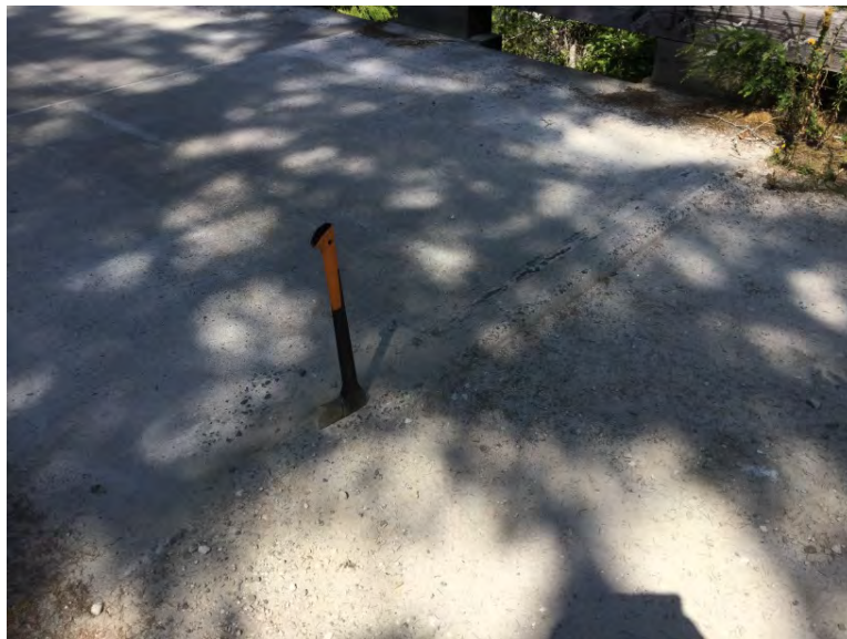
Ballast wall and first deck panel wearing
