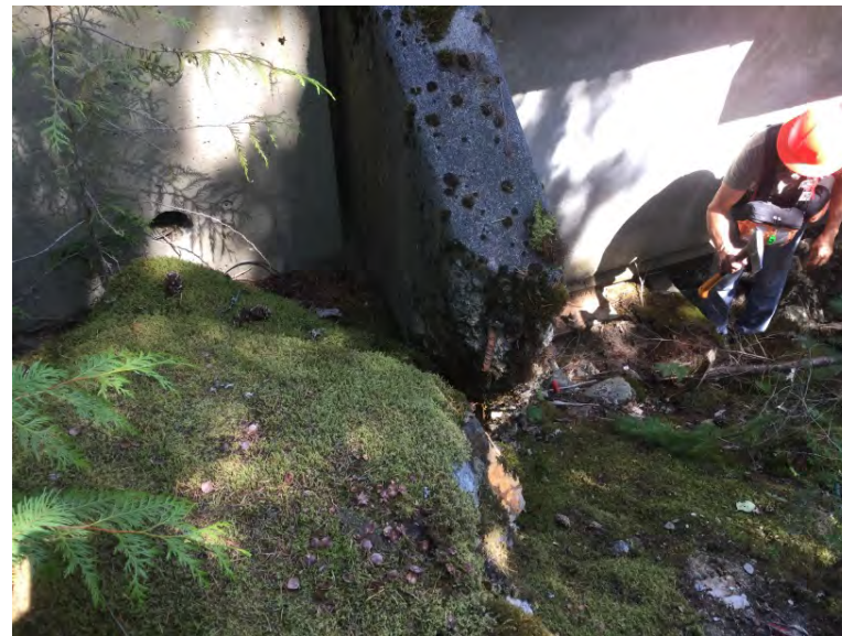
Ballast wall right bank upstream
