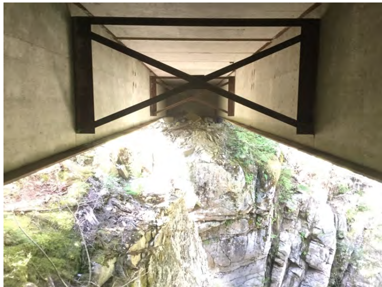
Approach from Right Bank when facing downstream
