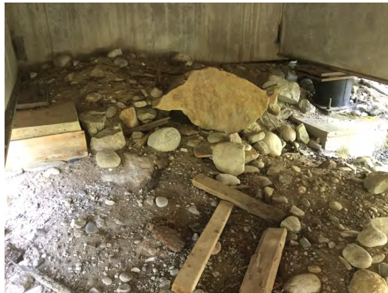
CIP footings at right bank
