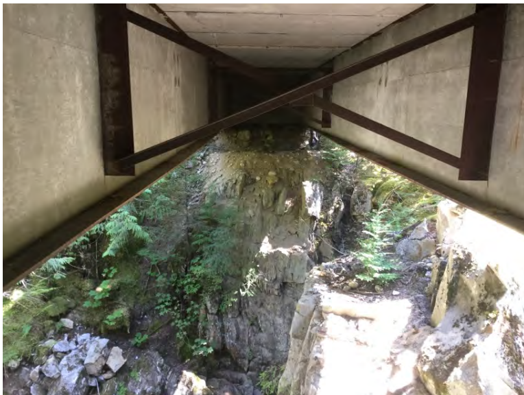
Left Bank Abutment when facing downstream
