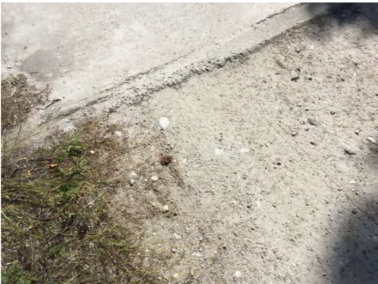
Wearing top of ballast wall right bank
